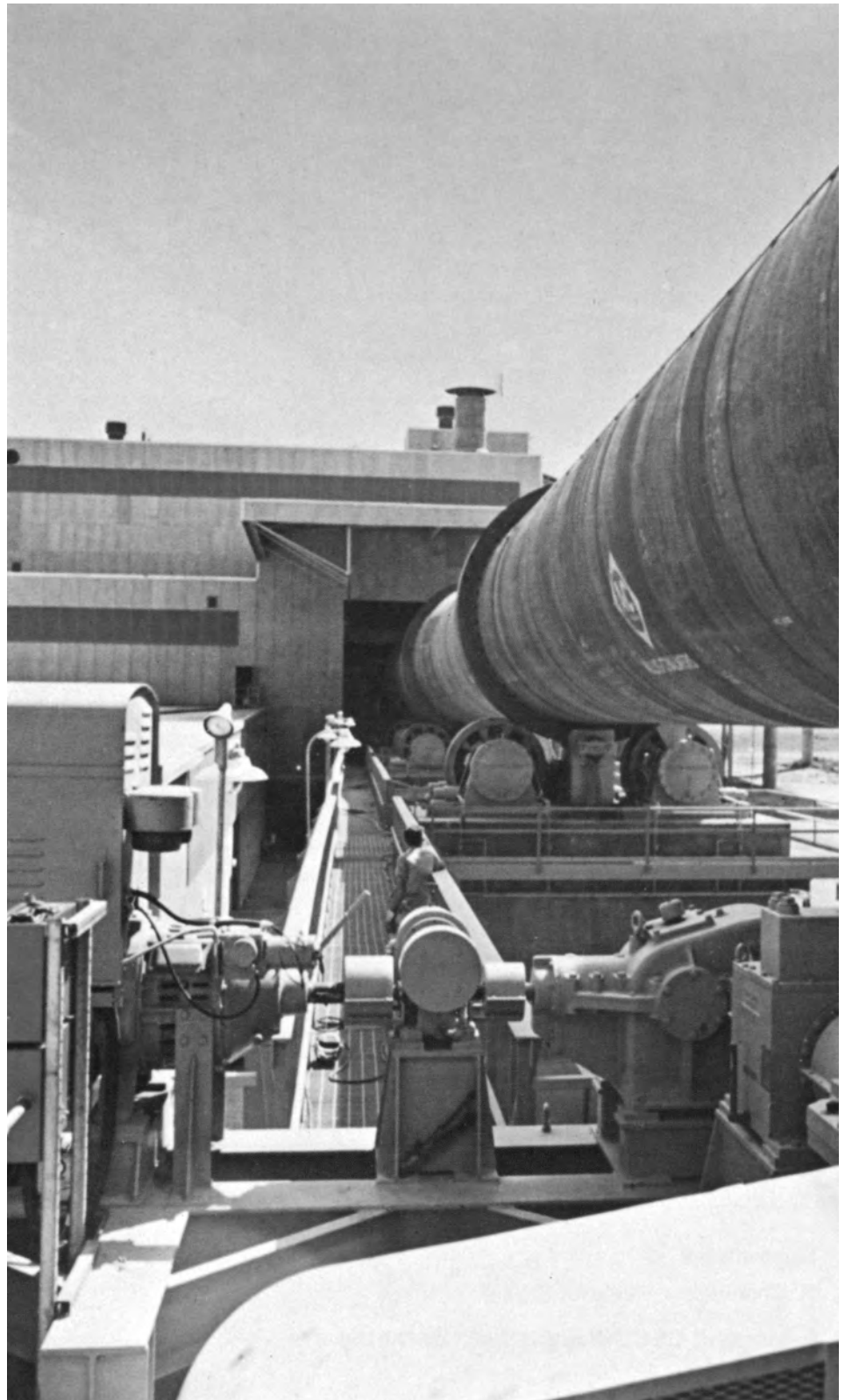
Photo: Marland CECON clutch and CEBMAG Backstop on modern cement kiln provide for emergency drive rotation in case of main power shutdown.
